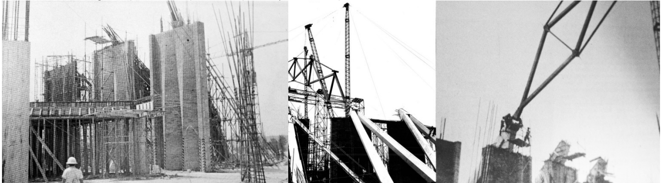
Figure 6. a) Folded walls; b) Buttresses; c) Assembly of the arches. (De Pablo, 1968; Murad Silva, 1967; Villasana Suverza, 2015).
