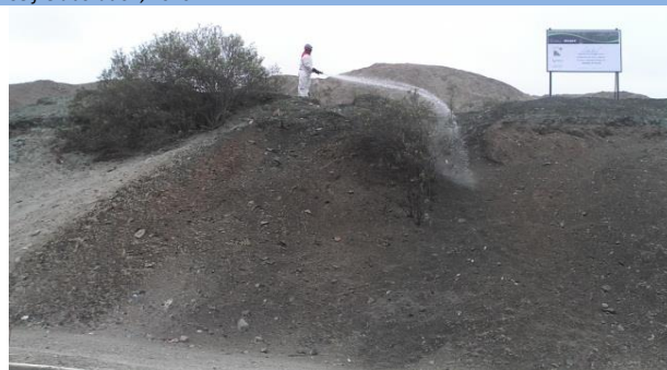
Figure 5. Applying particulate matter abatement product on slopes. Source: Self-elaboration, 2010.
