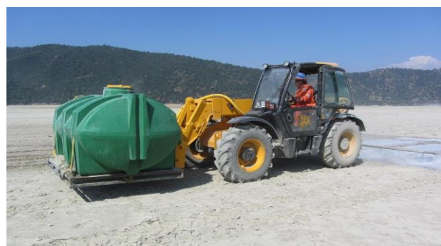
Figure 4. Applying particulate matter abatement product in areas with low bearing capacity. Source: Aguasin Ltd.
