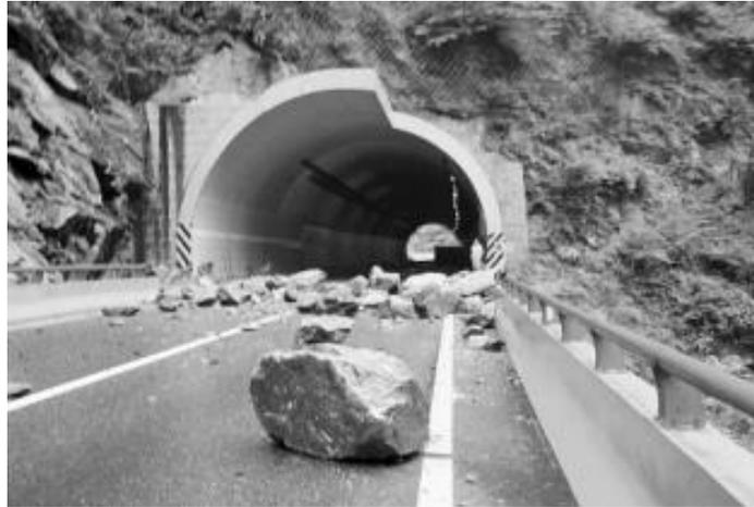
**Figure 1.** An example of rock fall event occurred on concrete tube (Hu et al. 2018).
