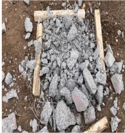
Figure 29. PCC slab after explosion with 250 g TNG.
