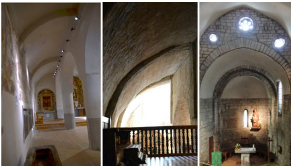
Figura 2. Bóvedas convexas funiculares Santa Eularia d'Unha (c. XII), Santa Maria d'Arties (c. XII-XIII) y Era Purificacio de Bossost (c. XII-XIII)
