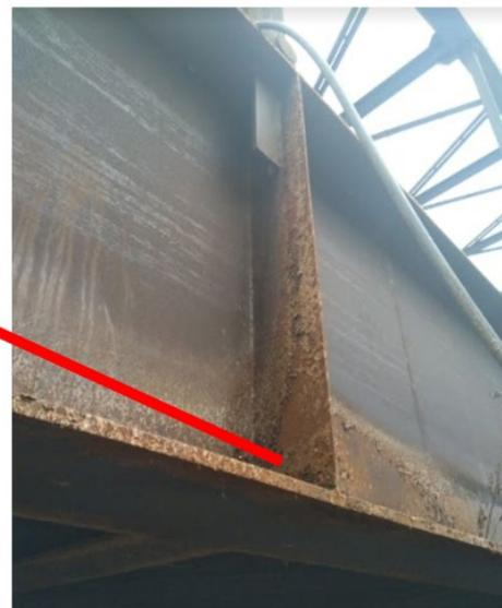
Figure 6. Oxidation and corrosion evidence found on the web stiffener of the main girder element of the Unete steel arch bridge
