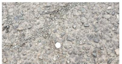
Figure 13. Surface damage for CDD=154.593 °C-days
