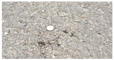
Figure 12. Surface damage for CDD=80.498 °C-days
