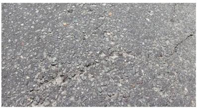
Figura 11. Surface damage for CDD=74.112 °C-days
