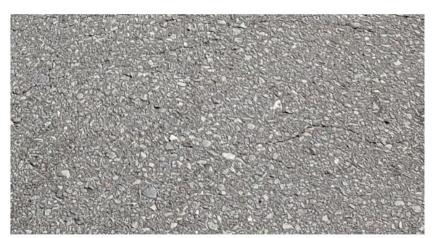
Figura 10. Surface damage for CDD=51.482 °C-days
